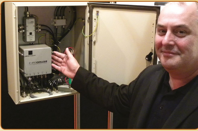
■ New at Globallnvacom: a housing with four stacked ODU32 components that provides eight identical optical connections, capable of feeding 256 points.
