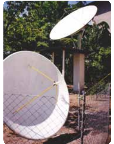
■ The small 1.5-meter dish in the foreground is used by Cahit to receive ASTRA 2 at 28.2 east
