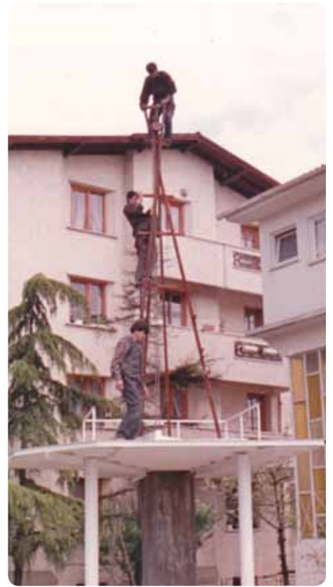
■ The mounting frame is being prepared
