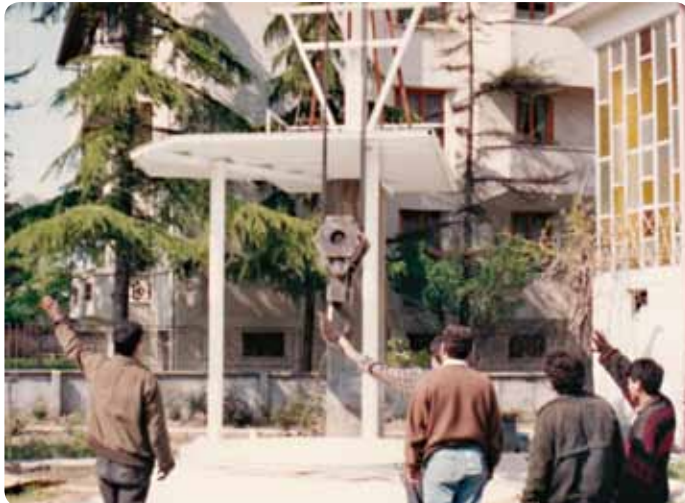
■ The crane lifts the dish in place
